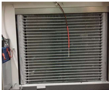
Figure 42. Replacing Exterior Cabinet Sensor Group
