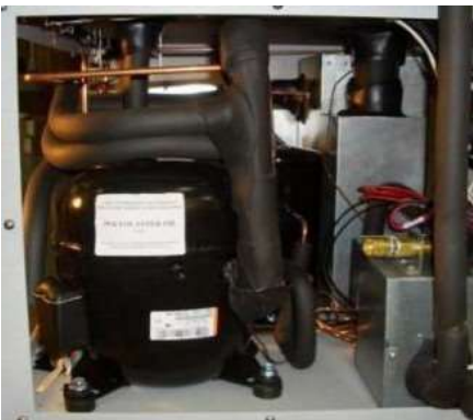
Figure 52. Replacing the Compressor
