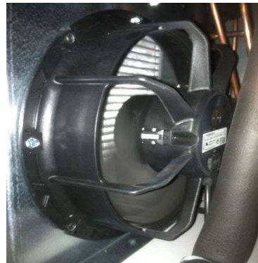
Figure 51. Condenser Fan
